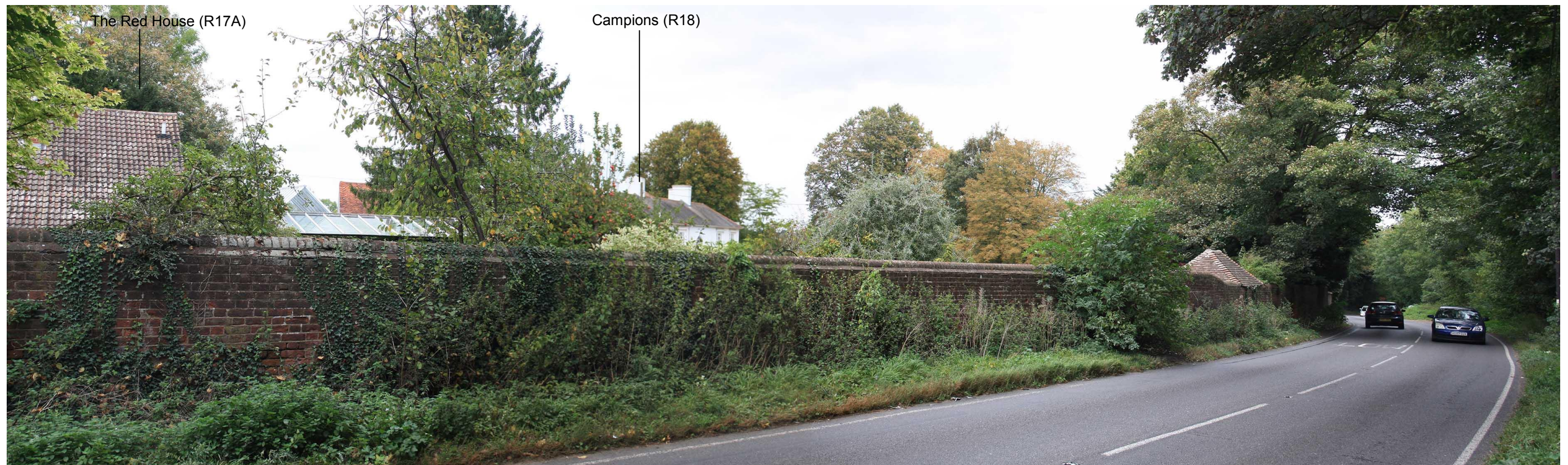
View 6: Sheering Road looking north. The road would be realigned eastward to join the proposed roundabout and link to the M11. The existing road would be downgraded & narrowed for residential access. Most of the trees to the right and all to left would be retained.
