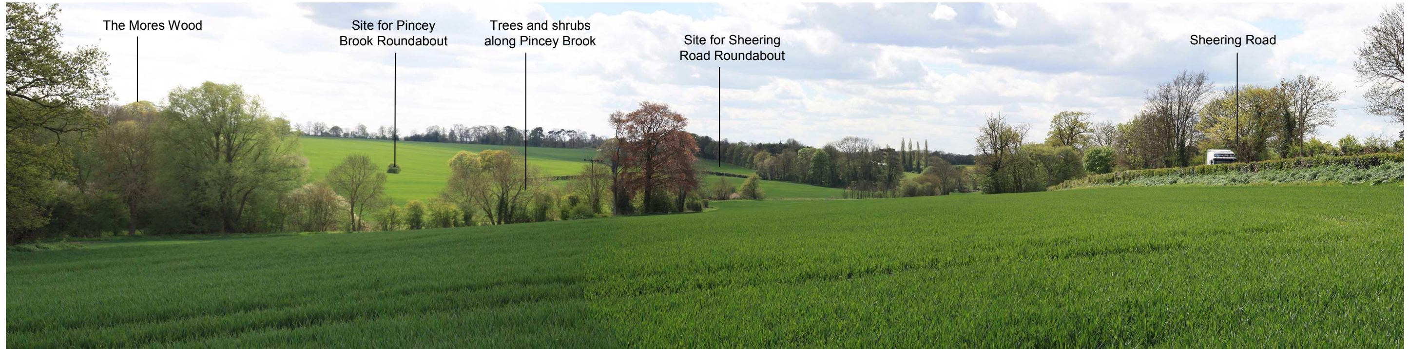
View 1: From rear of Sheering Hall Cottages (R23) across valley of Pincey Brook toward the site for the Pincey Brook and Sheering Road Roundabouts and proposed link roads.
