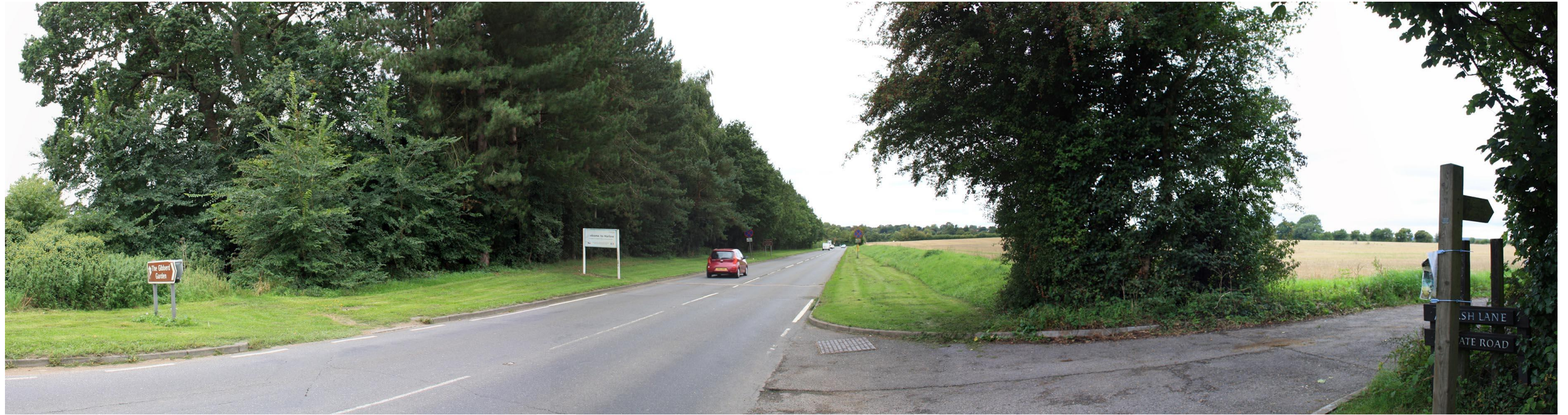
View 14: Gildden Way looking south. The turning on the right is Marsh Lane leading to the Gibberd Garden. The farmland to the right is included in the Harlowbury Development soon to start construction. Gildden Way road widening would encroach slightly on the belt of trees on the left side of the road and remove the tree clump in the foreground on the right. Noise barriers are proposed both sides of the road, next to the wood and along the boundary with the Harlowbury Development.
