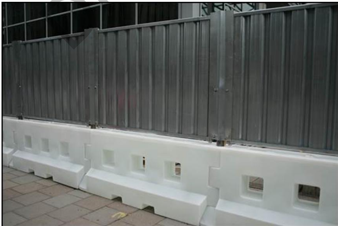
Water-filled Hoarding System
